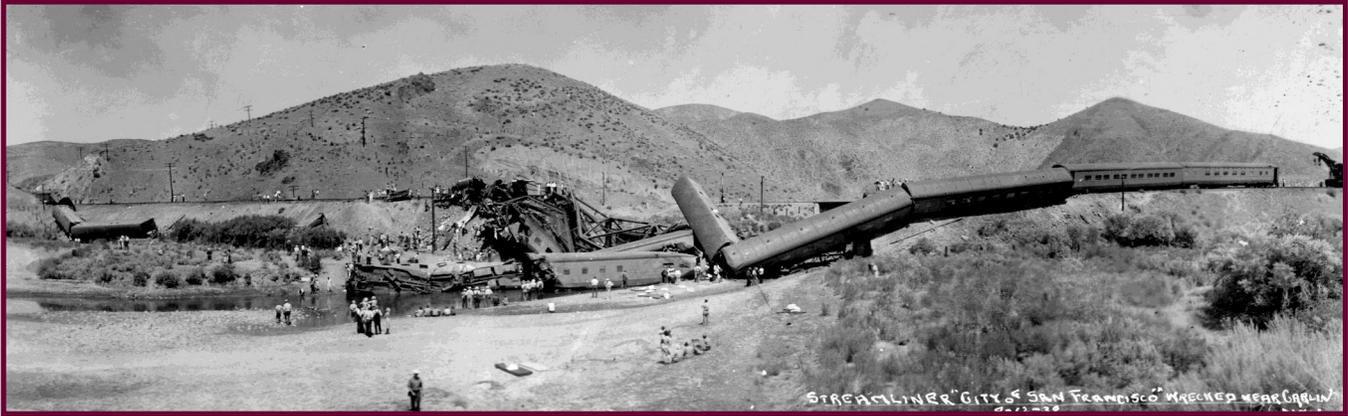
(Above) A northwestward panorama of the wreck on the morning after the derailment. Three diesel-electric locomotives and the first two train cars are to the left; the principal pileup of cars and bridge components is in the center of the scene. Trailing cars are to the right. L. B. Hanneman photo, NSRM Collection.
