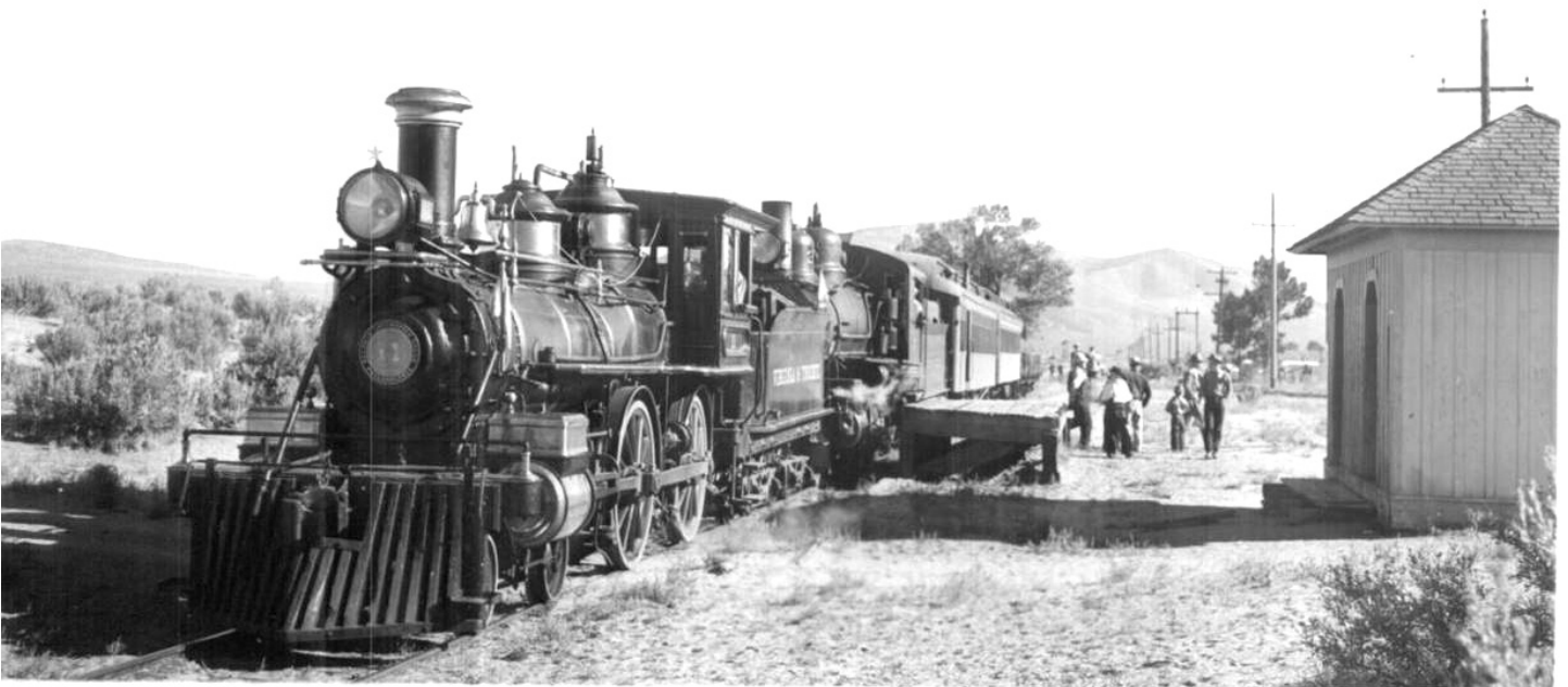
V&T No. 11, Reno, at Stewart shelter, 1949.
