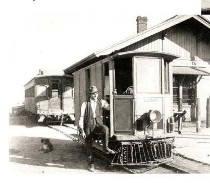
NC also owned a 4-cylinder 1928 Ford Model-AA 1½-ton truck that was never intended for rail service. After the wreck of No. 102, the NC shops rebuilt the truck in mid-1929 for rail passenger, baggage, and sacked-mail service as No. 107, NC's last motor car. It and No. 103 remained in service until NC's abandonment. Most of the railroad's assets were sold to the Hyman-Michaels Co. for scrap.
